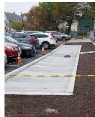
Construction of the concrete swale that demonstrates "grey" stormwater management
